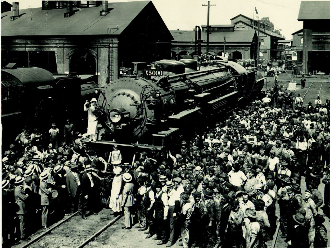
Figure 18. Celebration of the arrival of the Southern Pacific’s first 3-cylinder compound 4-10-2 class locomotive in the 1920s. In the background, from left to right: both ends of the Roundhouse (no longer extant), the Car Machine Shop, the Planing Mill, and the northwestern corner of the Erecting/Machine Shop, facing east.
