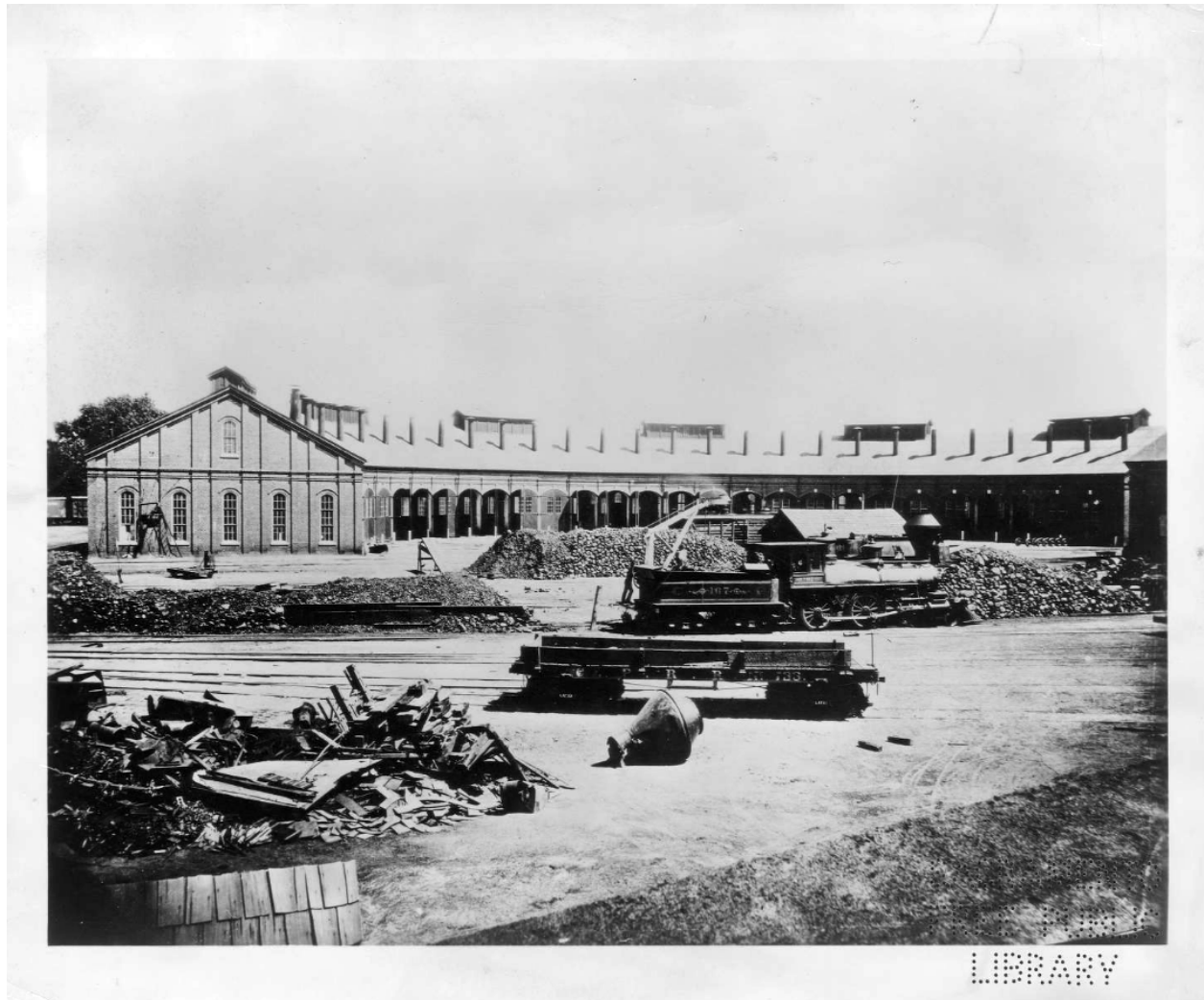
Figure 13. View of Roundhouse and Turntable, facing north (1874). The Roundhouse was removed in 1959 as part of the Southern Pacific Company’s transition from steam locomotives to diesel.
