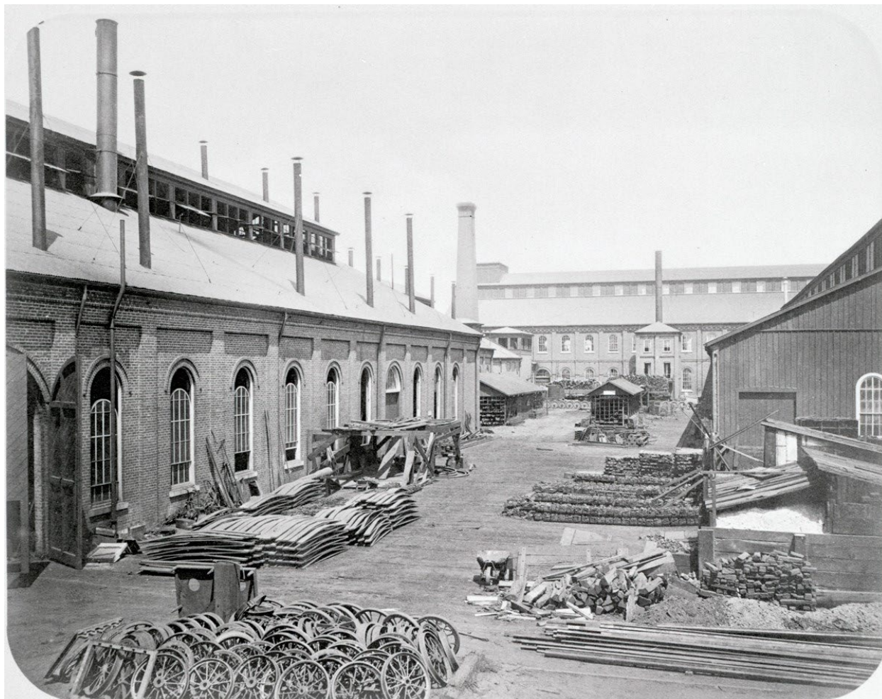
Figure 11. From left to right: view of Blacksmith Shop, Power House (no longer extant), Planing Mill, Privy, and Car Shop No. 3, facing north (1870s). Note the original brick walls of the Blacksmith Shop and the board-and-batten-clad southern wall of Car Shop No. 3.
