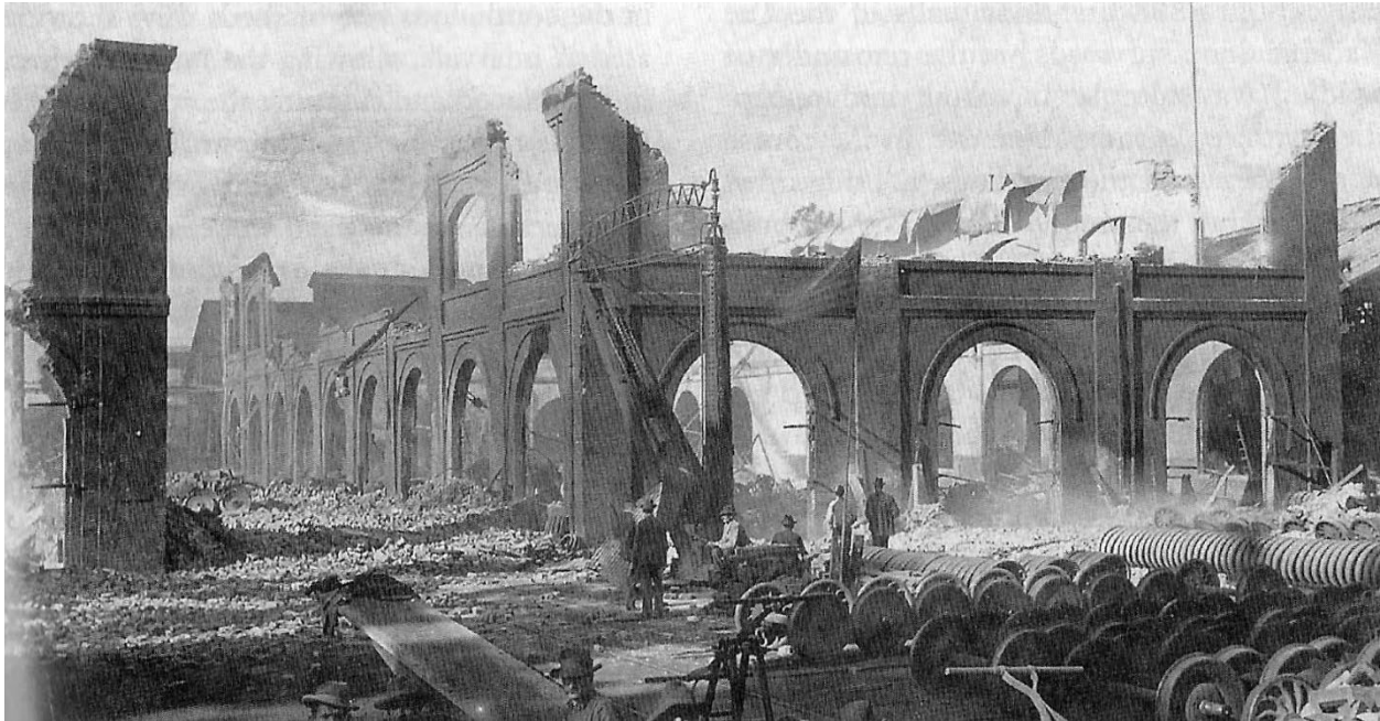
Figure 15. Car Machine Shop following a major fire in November 1898, view northwest. The Car Machine Shop and Planing Mill were both impacted by the fire, which originated in the second floor of the Car Machine Shop. Both buildings were reconstructed on their original foundations by the end of the following year.
