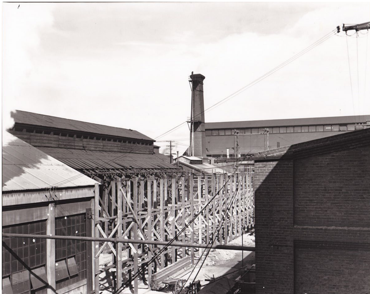
Figure 21. From left to right: view of Blacksmith Shop, Planing Mill, and Car Shop No. 3 (1939). The southern portion of the Blacksmith Shop had been renewed with reinforced concrete walls in 1929, and the addition to the northern portion is under construction in this photograph. The brick chimney of the Power House was removed in 1940, approximately one year after this photograph was taken.
