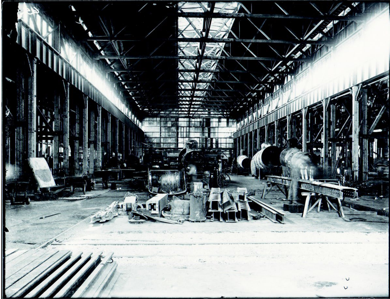
Figure 19. View of Boiler Shop interior during the steam era (undated).
